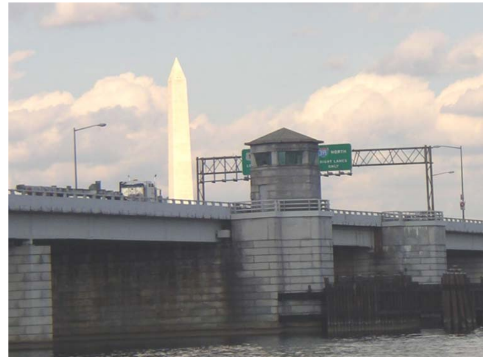
Photo 4 – Attendant Tower on the East Side of the Arland D. Williams Bridge.
