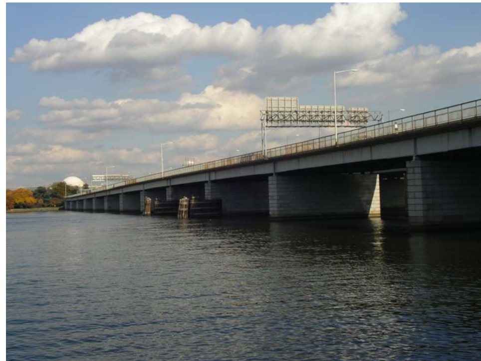
Photo 2 – George Mason Memorial Bridge
