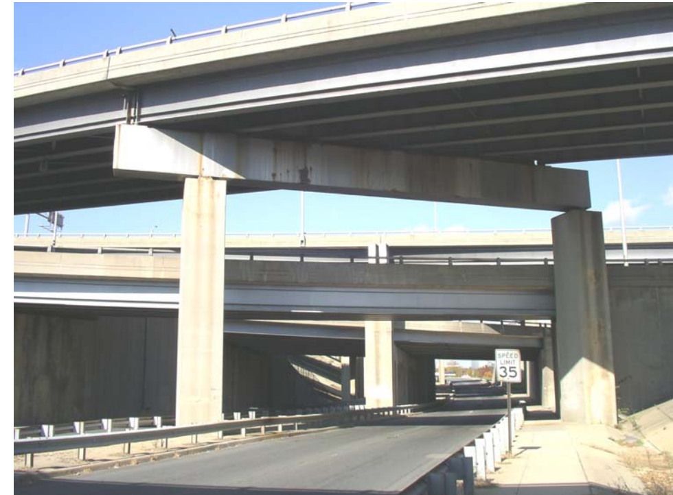
Photo 7 – Northern VA 27 Interchange at I-395 (Looking North).
