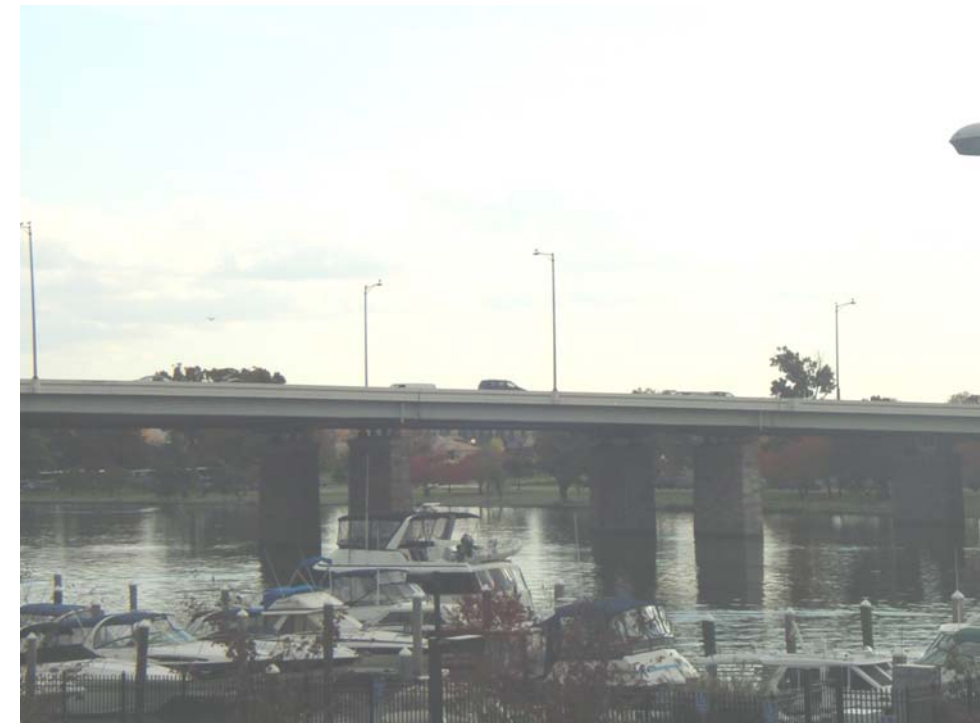
Photo 8 – North Elevation of the Francis Case Memorial Bridge
